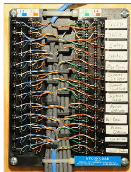
4-Line Phone Distribution via 110 punch down block
