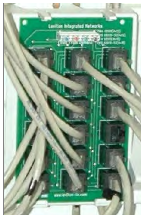
4-Line Phone Distribution via RJ45 distribution panel
